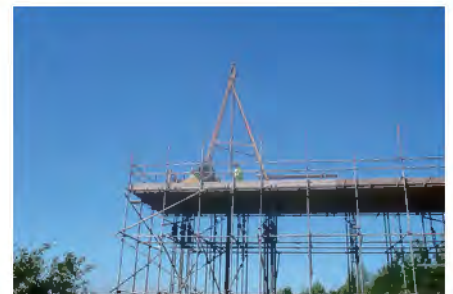
Working off a scaffold platform.
