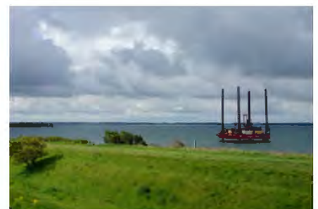
Aran 250 on site in Storstrom, Denmark.
