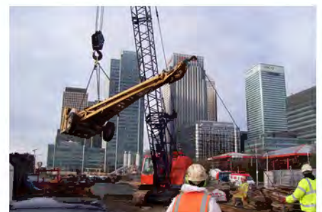
Craned to location.
