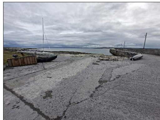
Photograph 4: View southeast of the entire slipway (centre) and pier (right) [RR; 14 Aug 2026]
