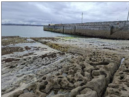
Photograph 3: View South of the existing slipway and pier in the background [RR; 14 Aug 2026]
