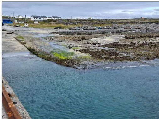
Photograph 1: View northwest of the existing slipway [RR; 14 Aug 2026]
