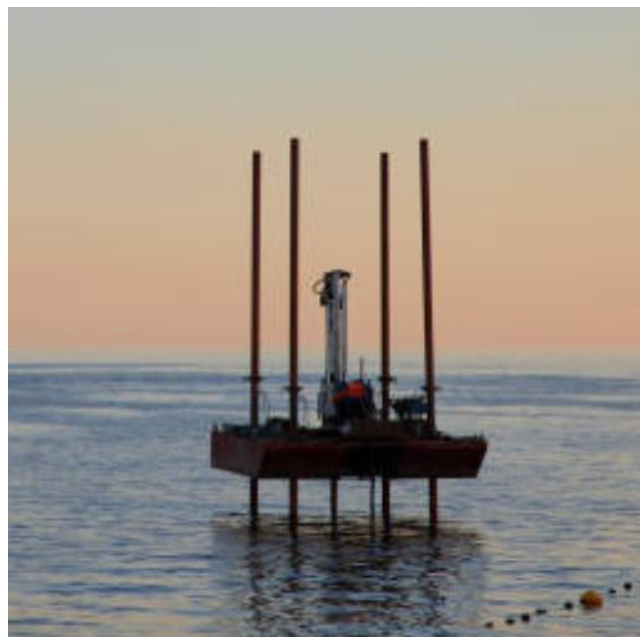
Figure 7. Example Jack Up Barge
