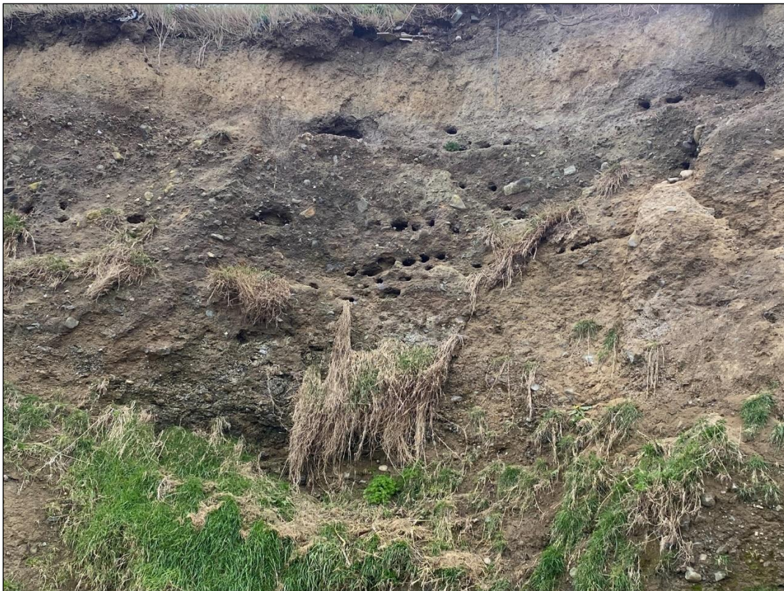
Figure D-2: Sand Martin burrows recorded in sea cliff adjacent to works area – 27-03-2025.
