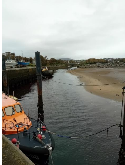
Plate 2. Looking east along the pier towards the Mill River. Dredge site. RNLI boat moored to the fore.
