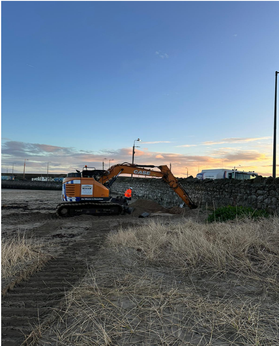
Figure 2-1: Image of excavator digging TP01
