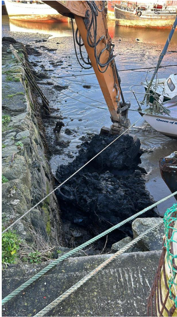
Figure 2-3: Grab sample being taken with excavator.
