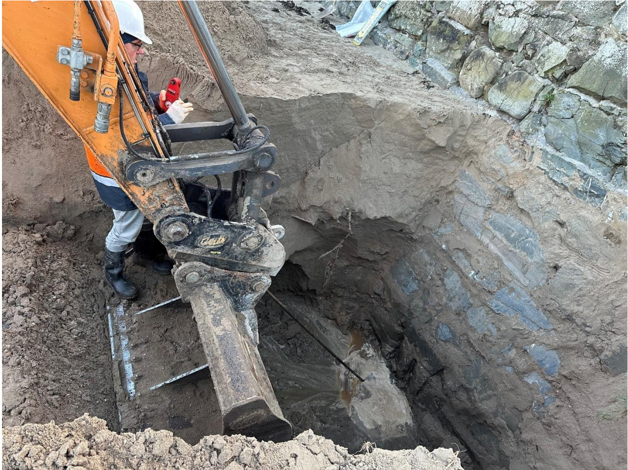
Figure 2-2: Hand vane testing being undertaken at TP01
