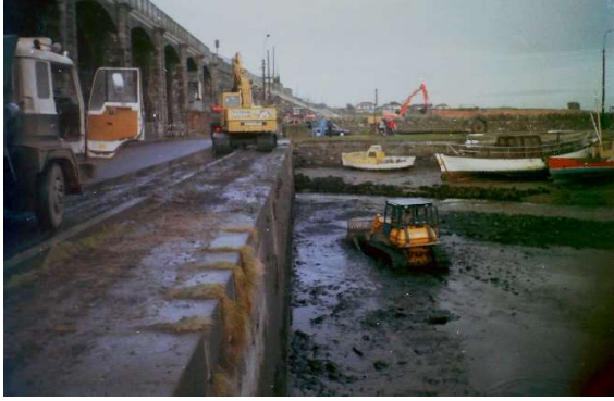
Figure 3-2: 1996 Dredging Campaign (Viaduct Walls)
