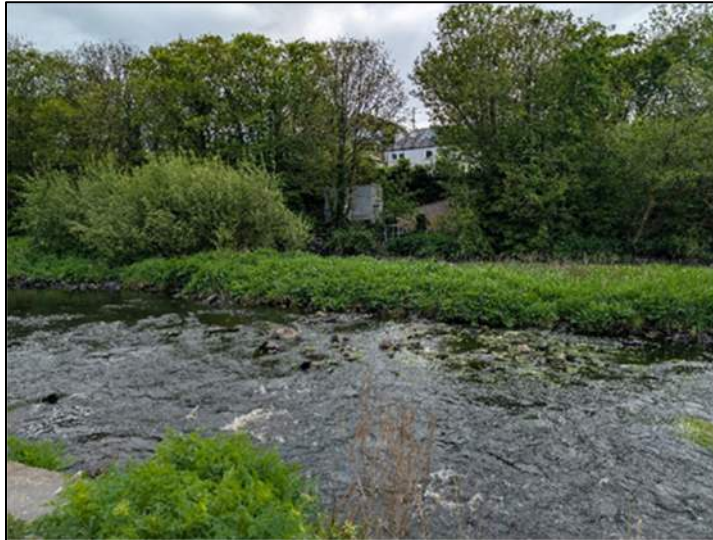
Photograph 7 – Existing foul water pump house infrastructure on southern bank [R.B. - 3/05/2026]
