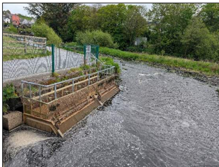
Photograph 6 – Intake/outfall and screen, possibly from hydroelectric power plant [R.B. - 3/05/2026]
