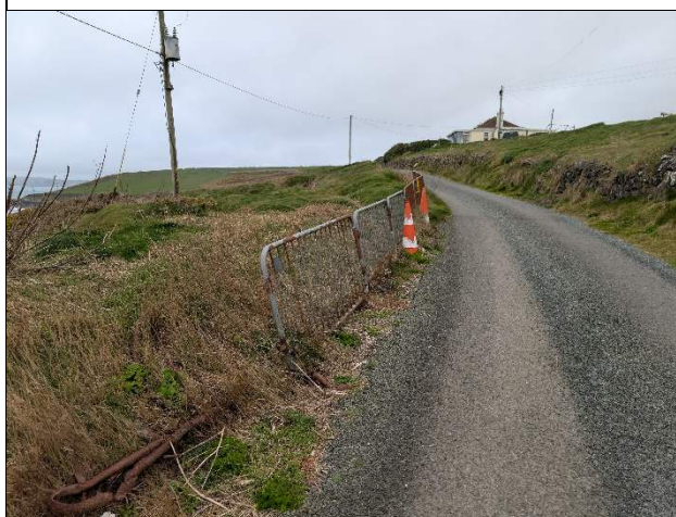
Picture 3: View West, subject area to left, barriers in place [RB: 16/03/2026]
