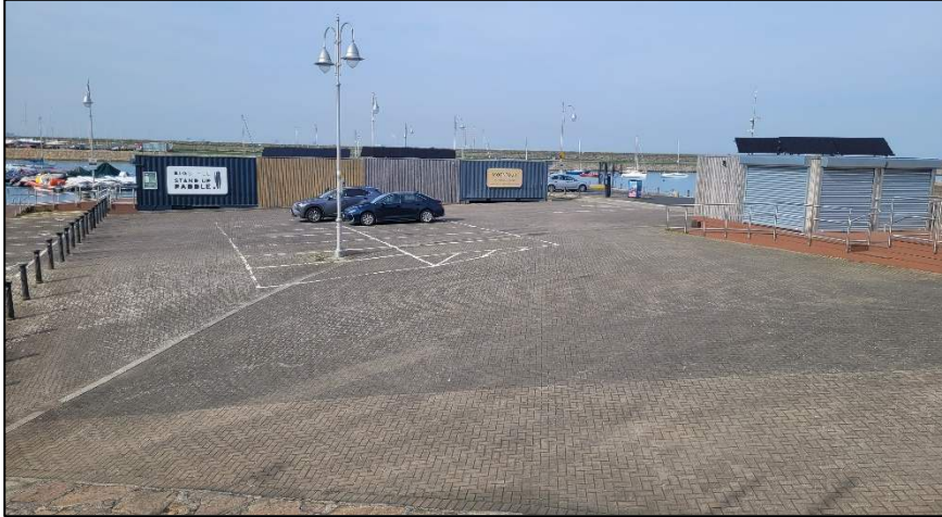
Photograph 2 – Looking southwest across the existing reclaimed lands at Area B with existing watersports business premises in background [PN 20/03/2026]
