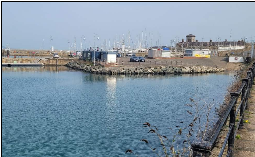
Photograph 3 – Looking east towards existing reclaimed lands at Area B bounded by rock armour revetment [PN 20/03/2026]
