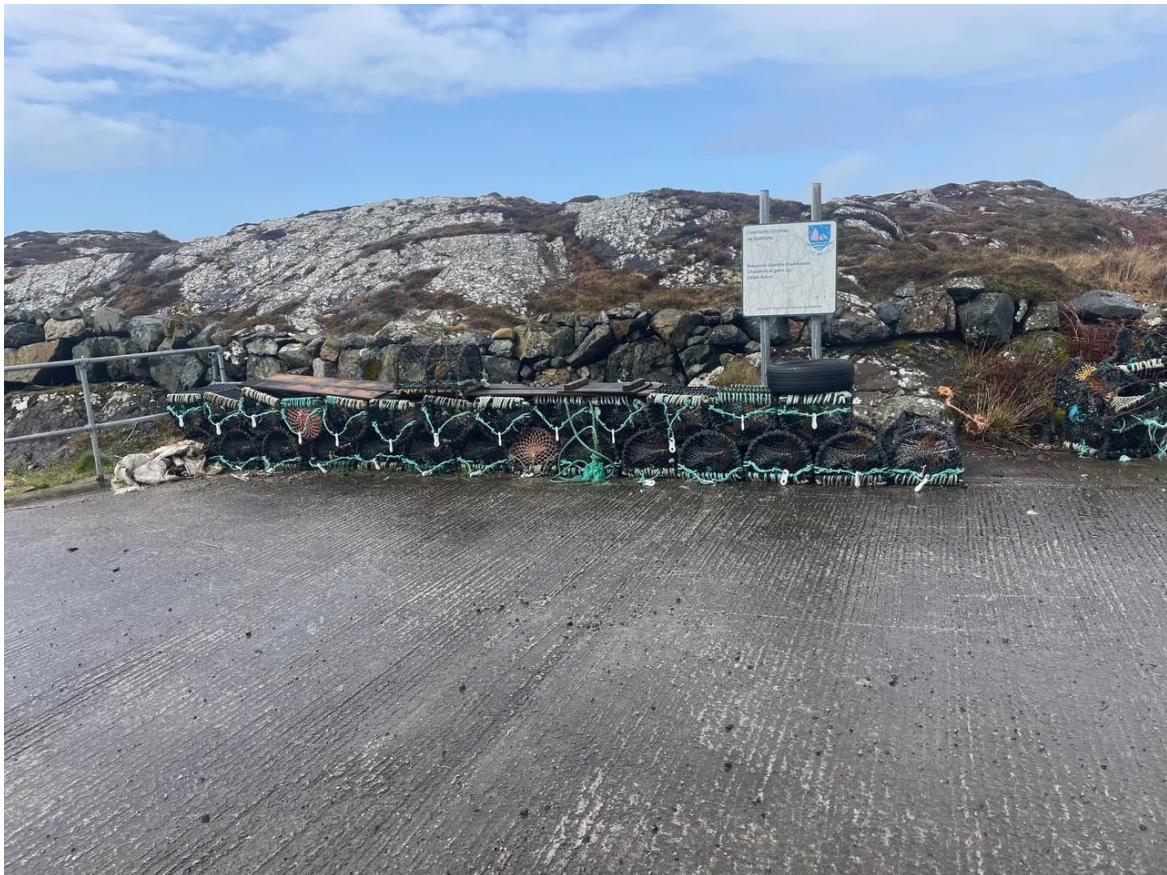
Photograph 3 - The existing pier (BMcD 24/03/2026)
