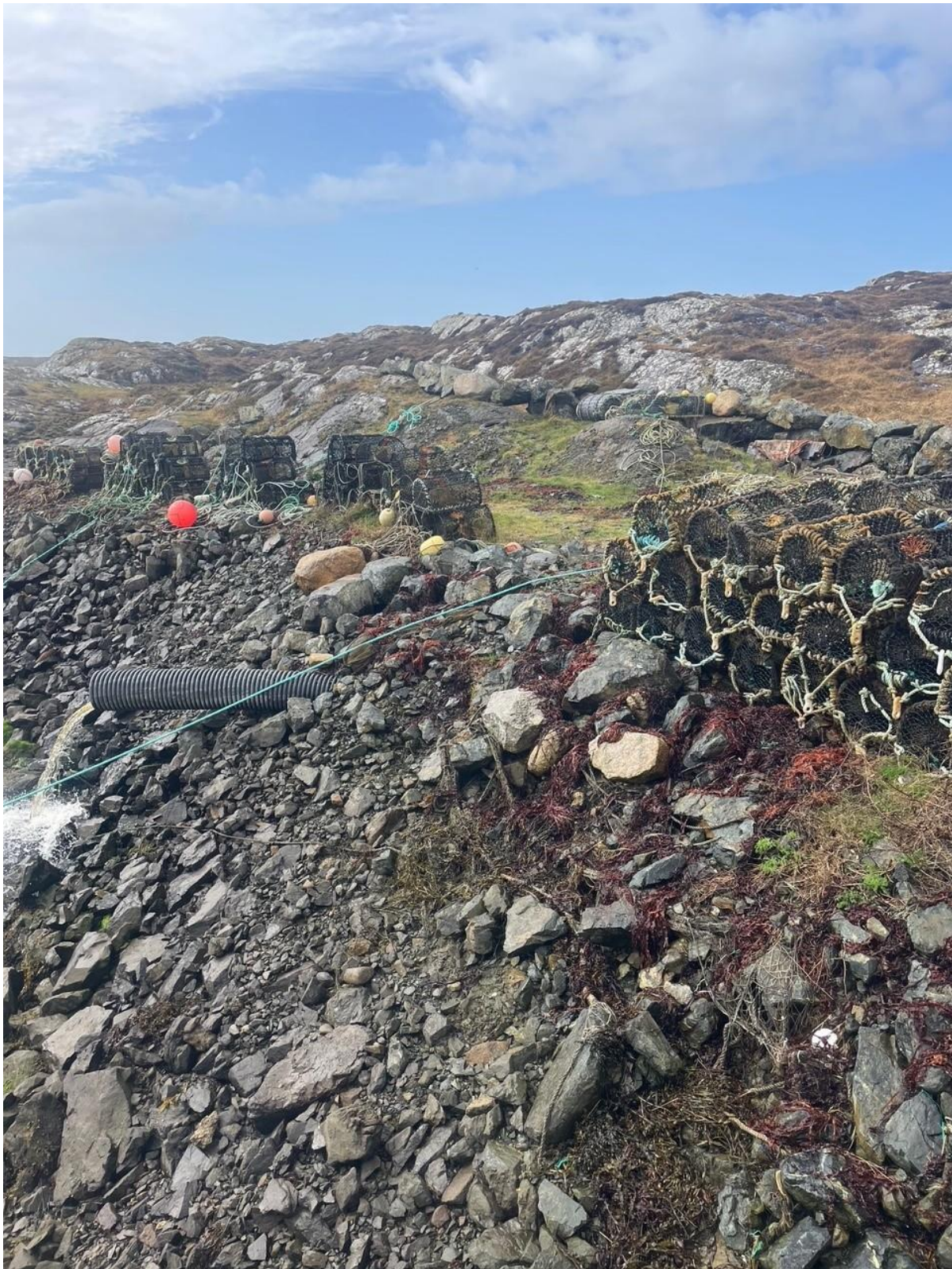
Photograph 5 - Site of pier extension (BMcD 24/03/2026)
