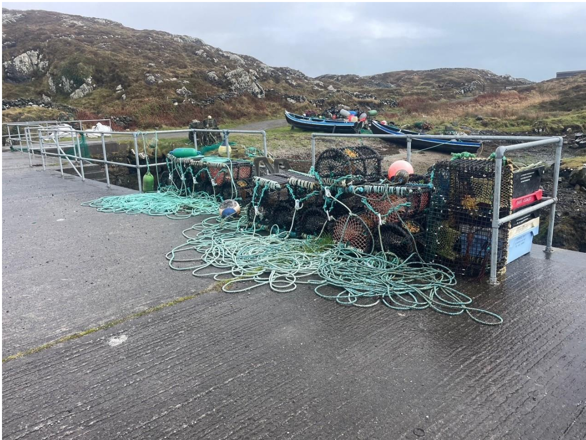
Photograph 2 - The existing pier (BMcD 24/03/2026)
