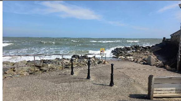
Photograph 2: Slipway adjacent to RNLI building [RR; 23 Apr 2026]
