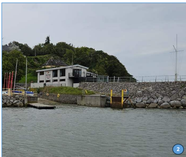
Photographs 2 & 3 – Rock Revetment and Reclamation Works to Northeast of Foynes Yacht Club (J.E. 06 09 2025)
