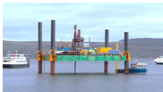
Figure 2.16 Jack-up Barge and drill rig
