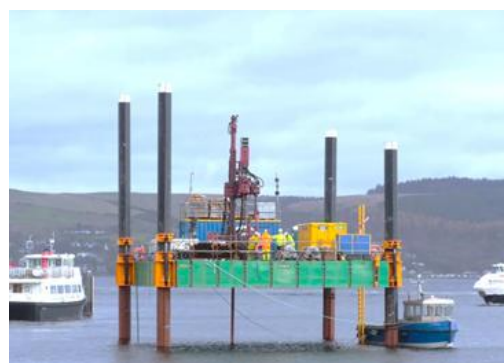
Figure 2.16 Jack-up Barge and drill rig
