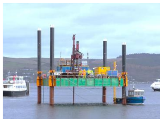
Figure 2-16 Jack-up Barge and drill rig
