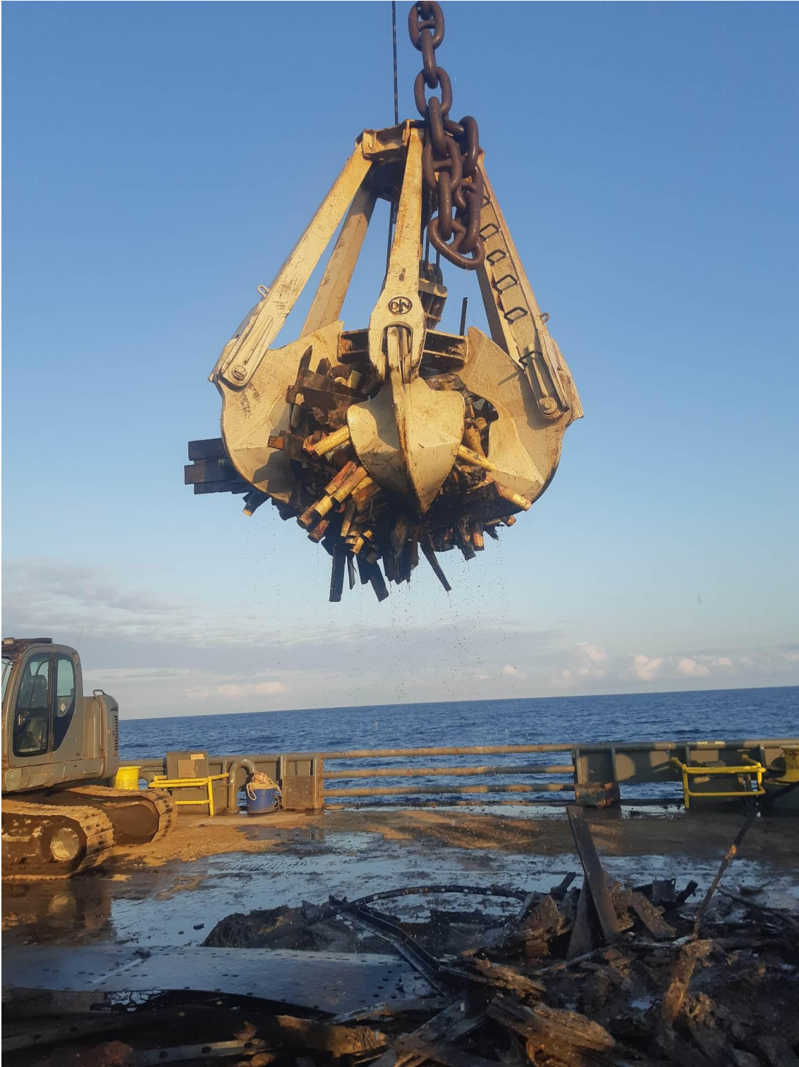
Figure A2. Camera/USBL-assisted mechanical grab returning commercial cargo to the N35. The method enables controlled vertical recovery without anchors.
