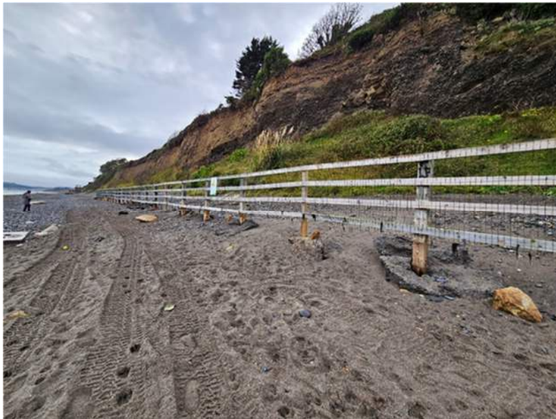
Photograph 5 – Area E showing sections of cliff erosion – [Mc.B. 26/11/2025].
