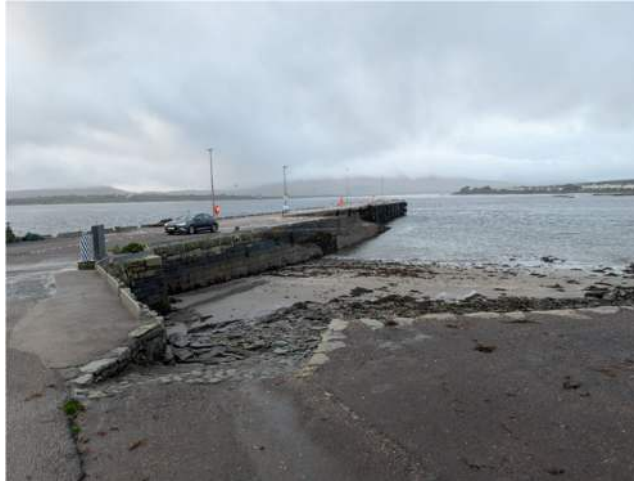
Photograph 4 – Overview of existing pier and slipway. [RB 4/11/2025]
