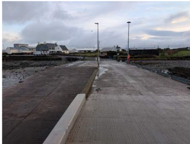
Photograph 2 – Access road and pier looking northeast. [RB 4/11/2025]
