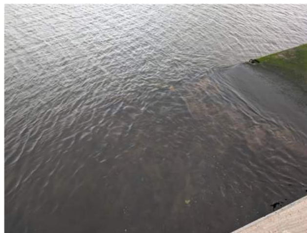
Photograph 3 – Toe of existing slipway. [RB 4/11/2025]
