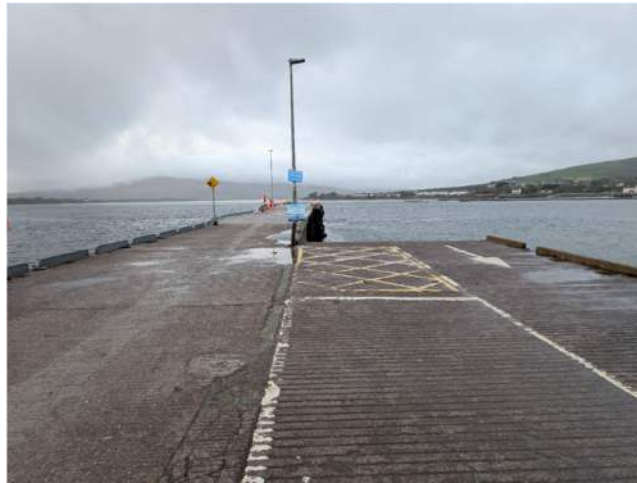
Photograph 1 – Access road and pier looking southwest. [RB 4/11/2025]
