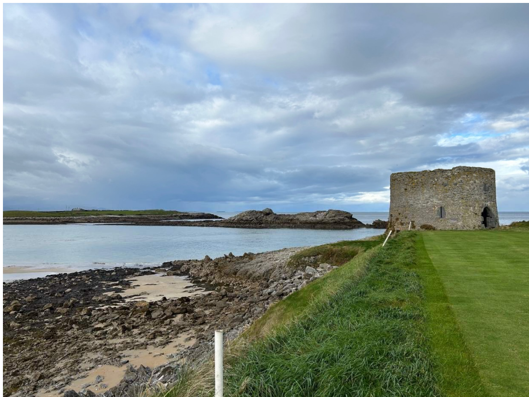
Photograph 2 – View taken from southeast looking northwest with Barrow Round Castle to the right
