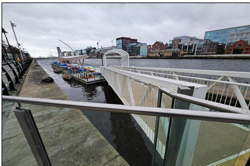
Photograph 2 - Existing Jeanie Johnston pontoons at Area B [J.McC 29/01/2026]
