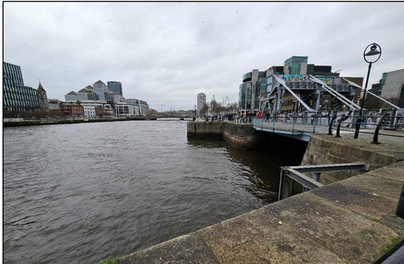
Photograph 1 - Existing access to George's Dock at Area A [J.McC 29/01/2026]
