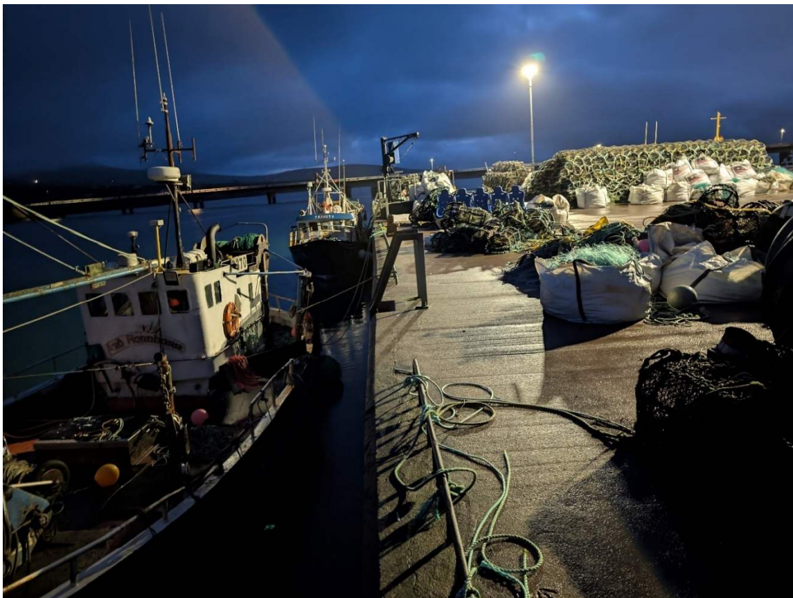
Photograph 5 – Head of Existing Pier (RB 4/11/26)
