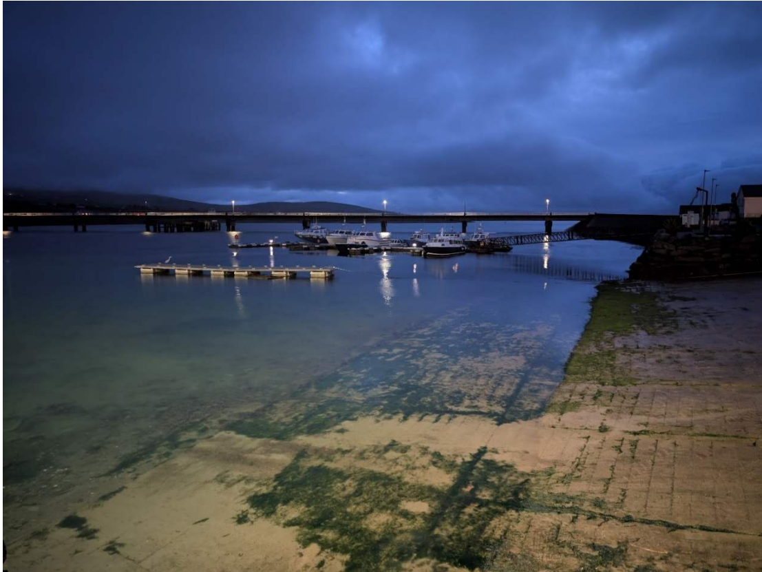
Photograph 1 – Area of proposed slipway extension, Applicant pontoons with boats in background with unauthorised third party pontoon evident in front and to the left. (RB 4/11/26)
