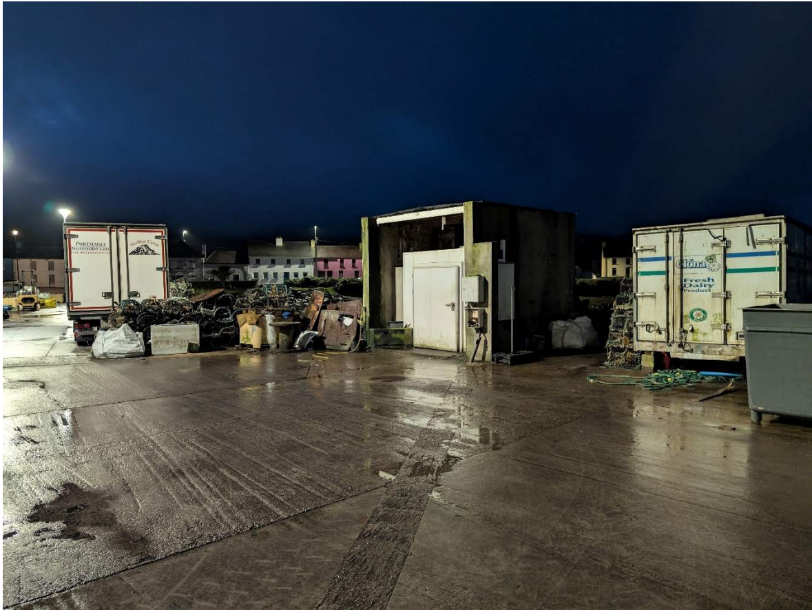
Photograph 6 – Ice plant on pier (RB 4/11/26)
