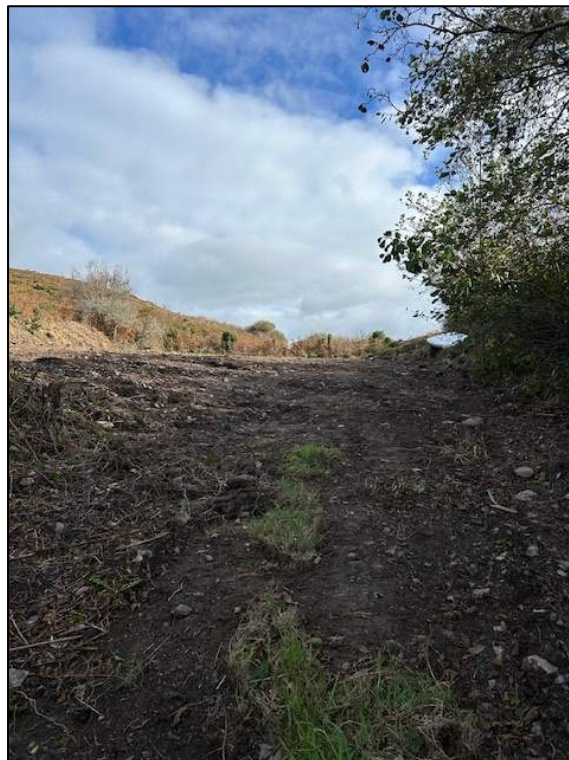
Photograph 3: View from launch site at Ringarogy looking east toward track leading to public road [NL 21 October 2025]
