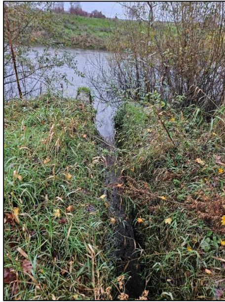
Photograph 5 – Area E of proposed MAC area; looking east [JMC 30 October 2025]
