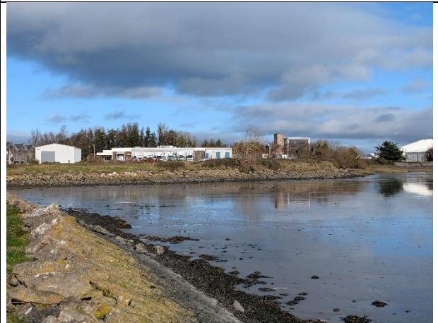
Picture 16: Area I from revetment, looking NW, RB
