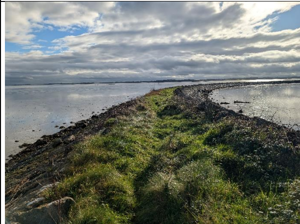
Picture 11: Revetment, Area I, RB
