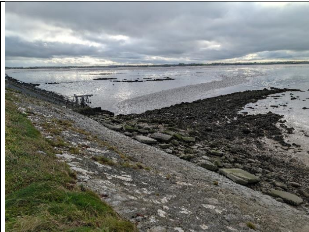
Picture 25: Area F, looking SE, RB
