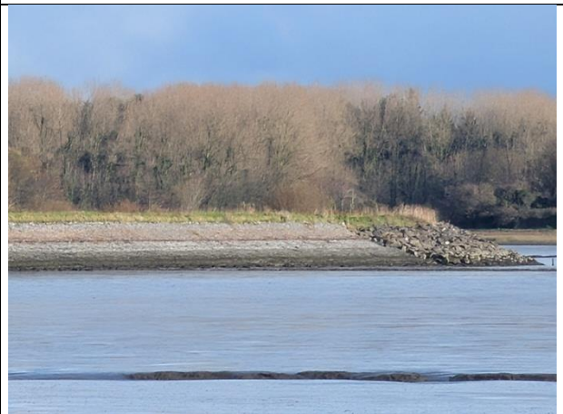
Picture 18: view NE from revetment toward Area J, RB
