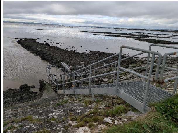
Picture 27: sluice access to shore, Area F, RB
