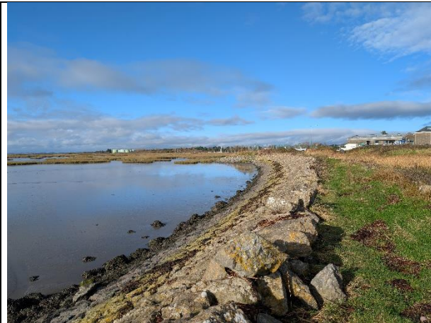
Picture 13: Revetment, Area I, RB
