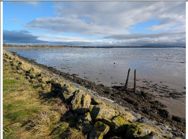
Picture 14: East side of revetment, Area I looking East, RB
