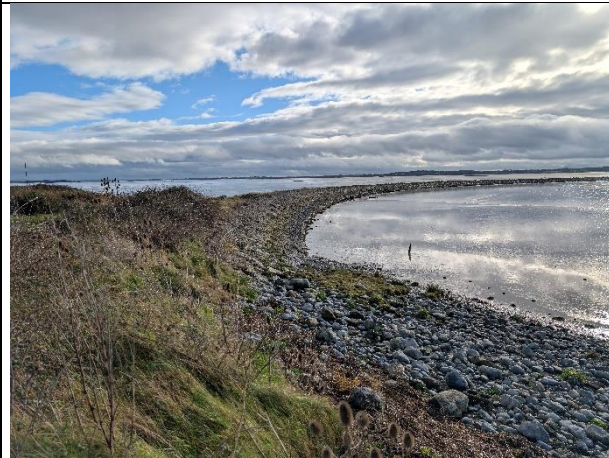
Picture 9: Root of revetment, Area I, RB
