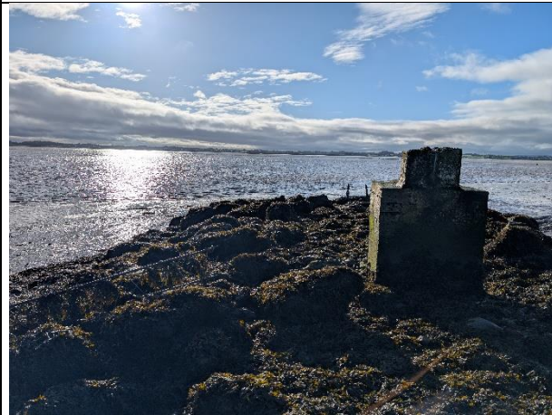
Picture 15: End of revetment Area I looking south, RB
