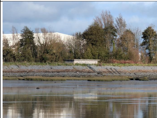
Picture 17: Shore access & facility located midway east of shoreline on Area I, RB
