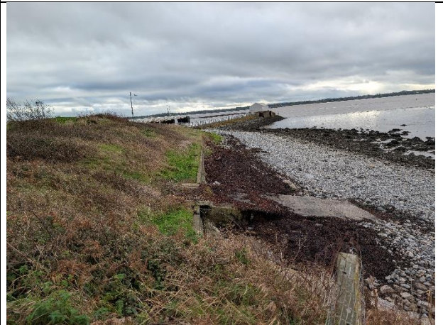
Picture 28: Area immediately South of MAC Area F, RB
