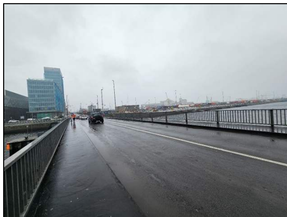
Photo 4 – View of existing Tom Clarke Bridge looking north [JM: 30 October 2025].
