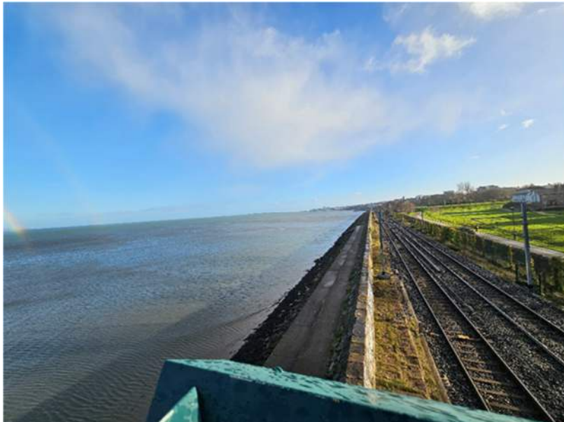
Photograph 5 – Existing pedestrian walkway in Area B at Booterstown looking South – [J.Mc. 28/11/2025]
