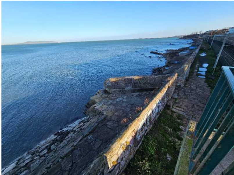
Photograph 7 – Area C and D Looking South at Blackrock Station – [J.Mc. 28/11/2025]
