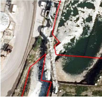
Figure 1 Aerial photography of bridge between Area B polygons
