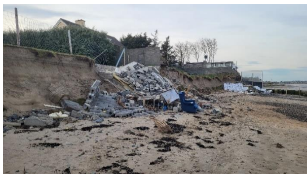
Photograph 4 – View looking north along beach with evidence of recent property damage due to ongoing coastal erosion [REDACTED] 4/03/2025]
