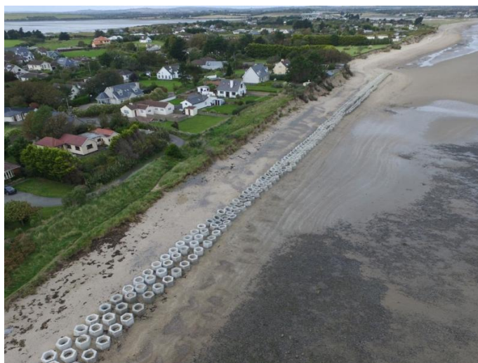
Photograph 1 – Existing 'seabee' units installed in 2018 (Copyright of Fingal County Council, sourced from Fingal County Council website)
