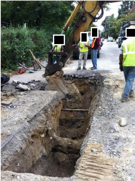
Figure 3.2. Slit trench example
