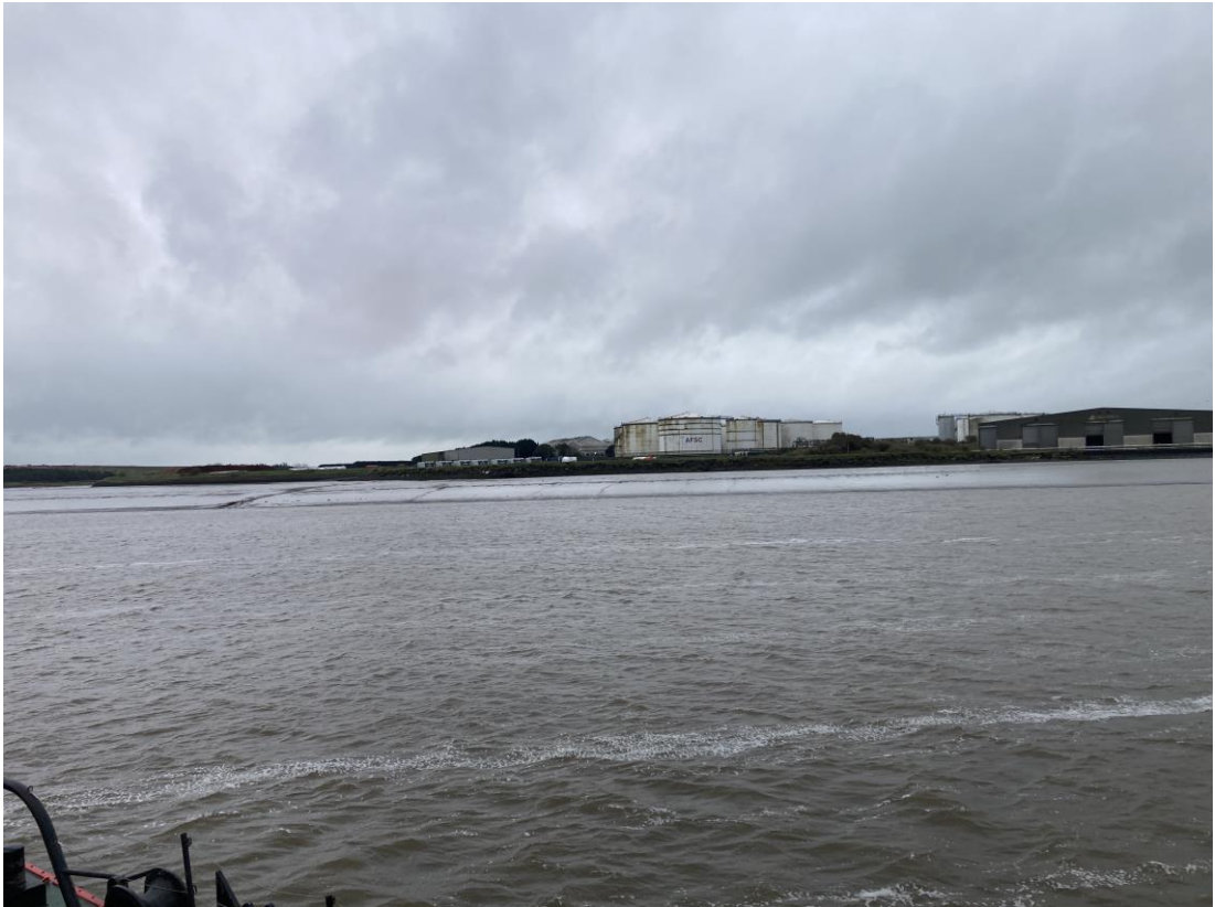
Photo 2 Site of proposed access bridge with SFPC Facility in the background (BMcD 26/03/2024)
